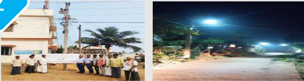
Street Lights installation work carried out-100No's
